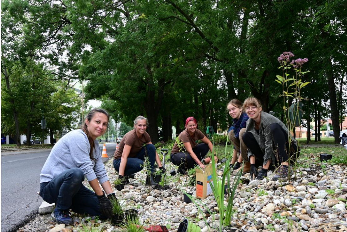
Fig. 4.20.4. The completed rain garden and the builders.
