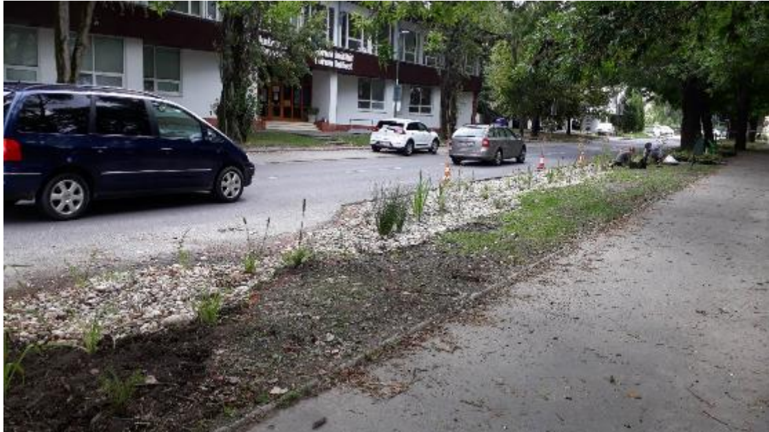
Fig. 4.20.5. The complete rain garden.
