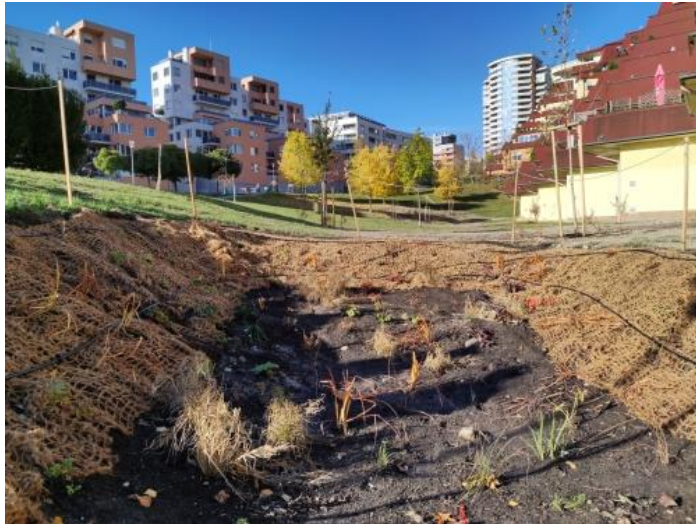
Fig. 4.19.3. The basin for the rain garden.
