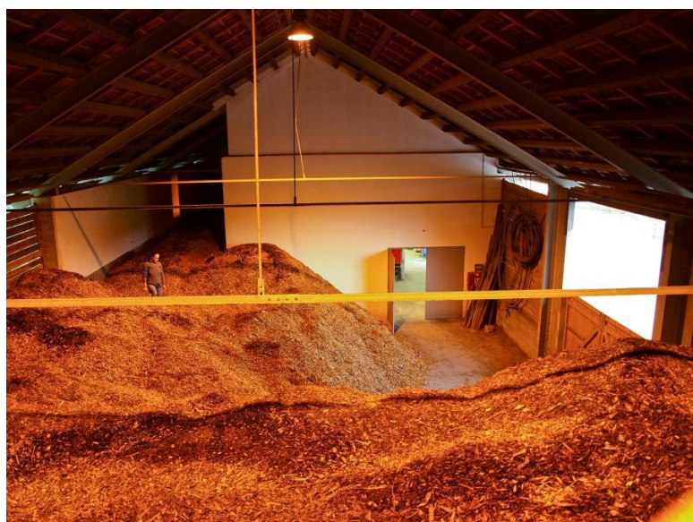
Fig. 4.4.2. Eco-friendly heating material in a storage.
