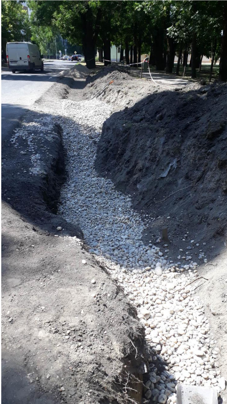
Fig. 4.20.3. Creating the rain garden.
