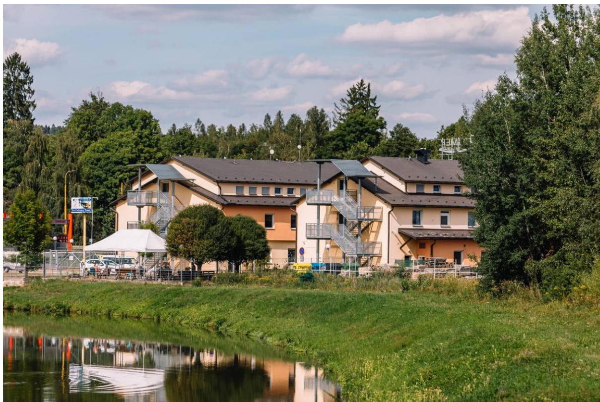
Fig. 3.3.3. Renovated and repurposed hotel in Czechia.
