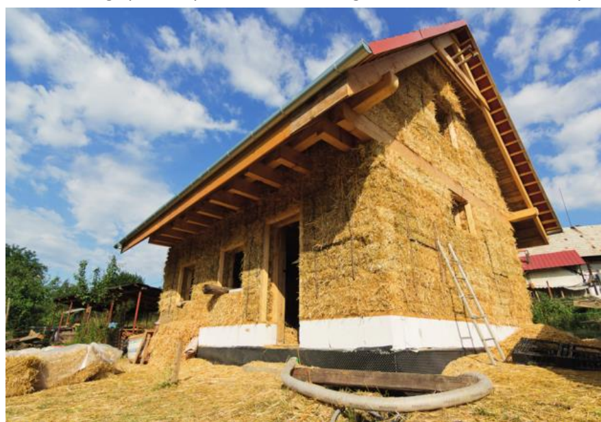
Fig. 4.9.2. Straw house as a passive building
