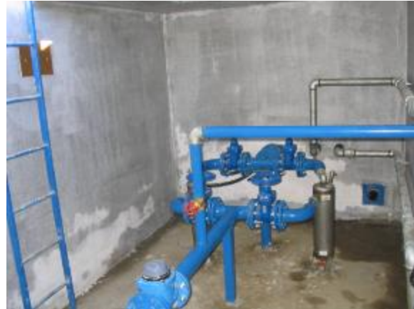
Fig. 4.15.3. Groundwater well providing heat.
