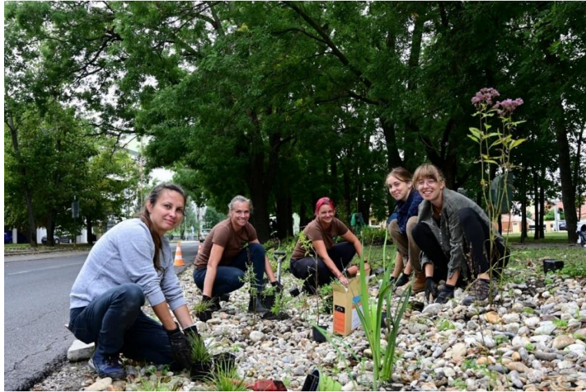
Fig. 9.4. The completed rain garden and the builders.
