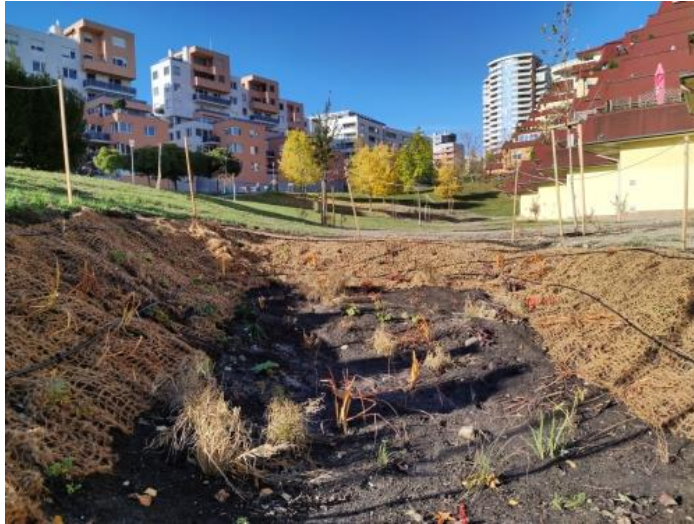
Fig. 7.3. The basin for the rain garden.
