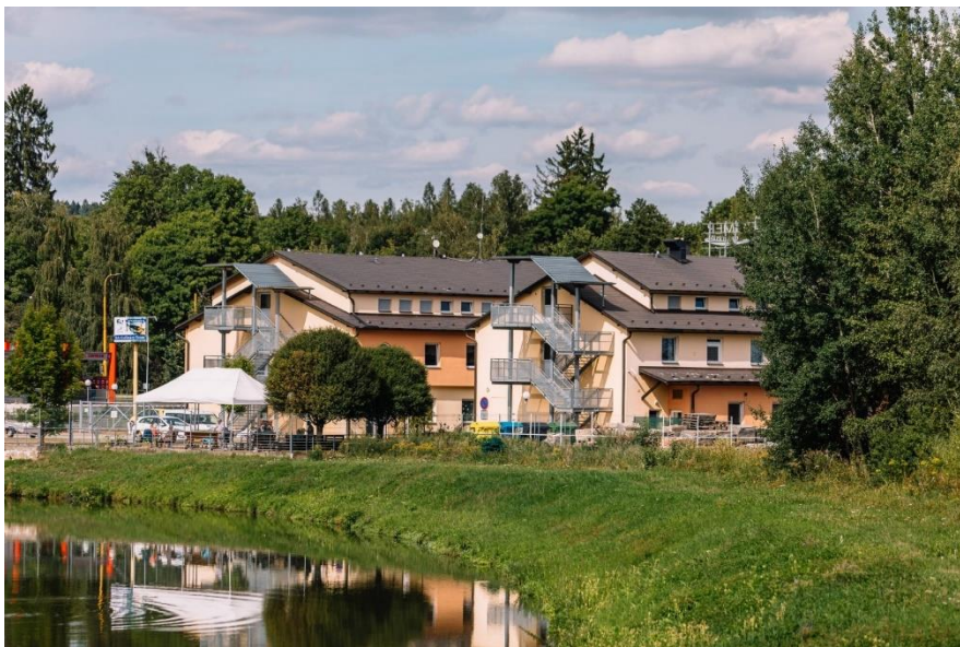
Fig. 5.3. Renovated and repurposed hotel in Czechia.
