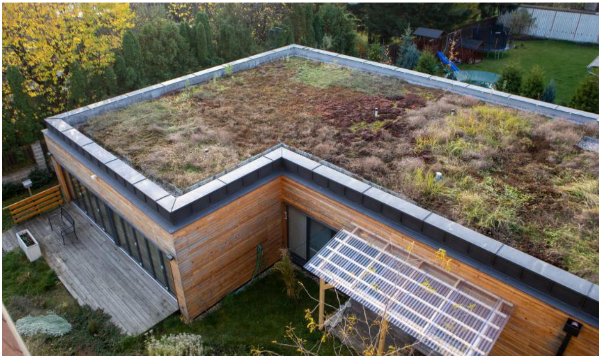
Fig. 6.3. Extensive green roof.
