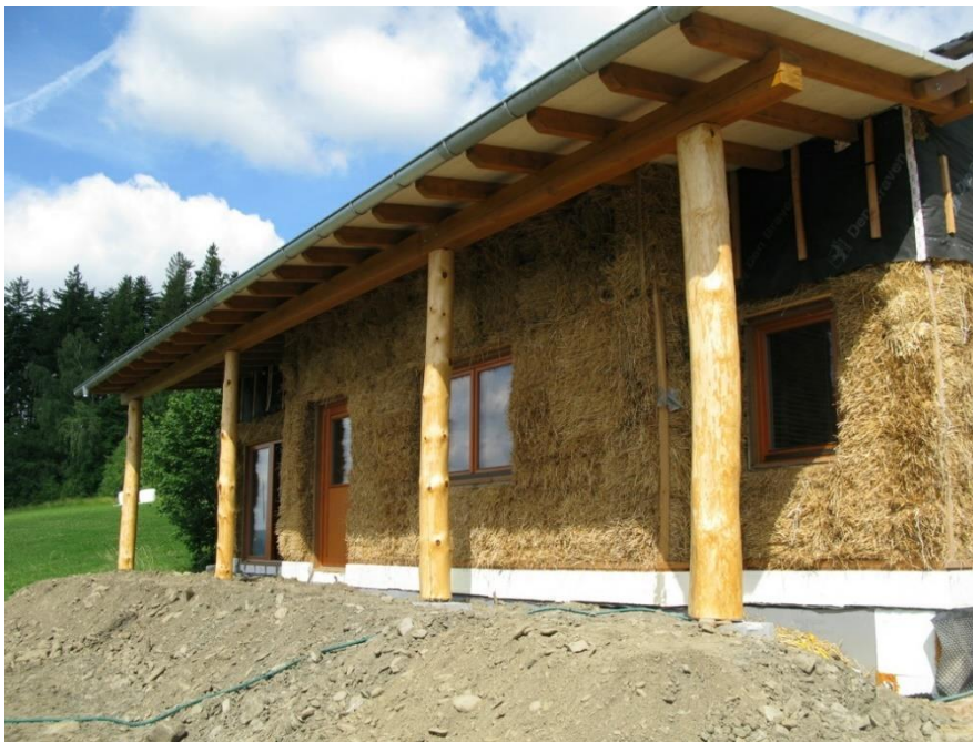
Fig. 9.3. Traditional design but innovative and green building method.
