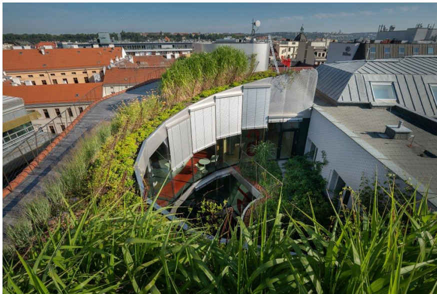
Fig. 3.3. Green roof and inner garden in Hostětín.
